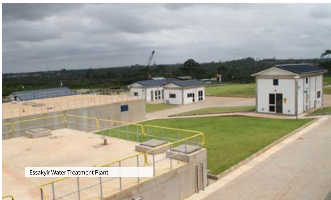
Five Towns Water Supply project
