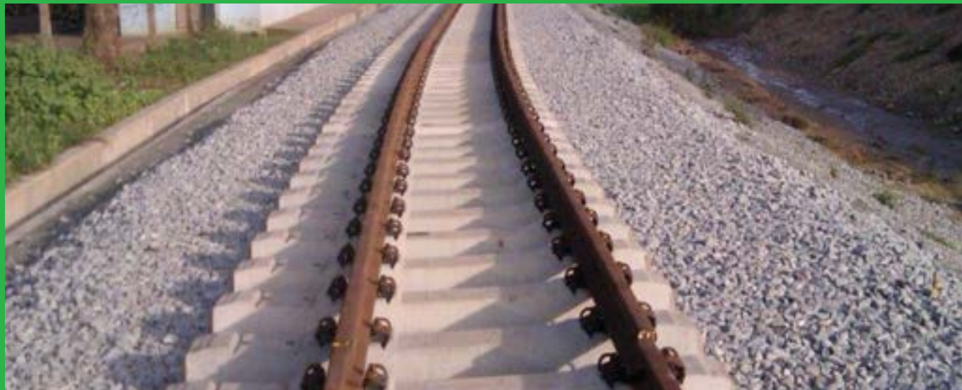
Newly completed Sekondi-Takoradi via Kojokrom Railway Line
